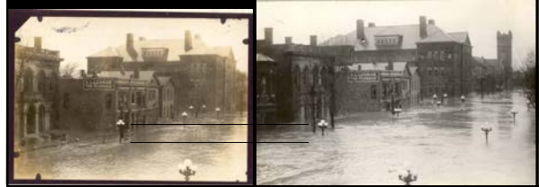
Lamp posts are ~13 ft high
